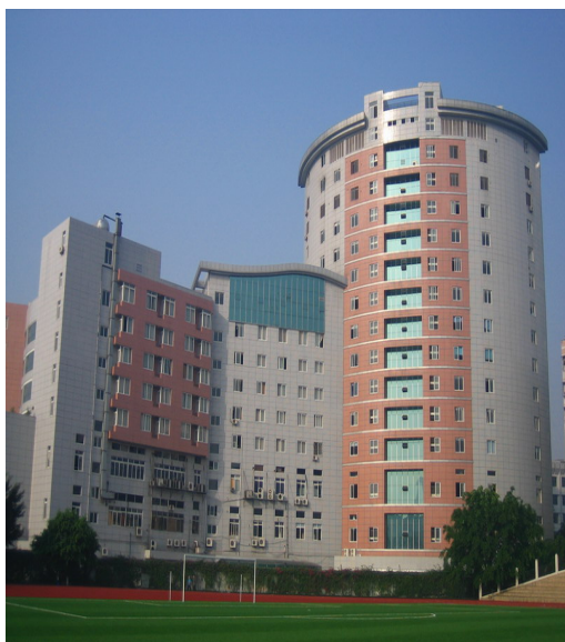
Class room Building
